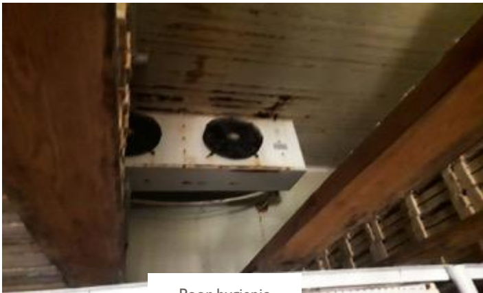
Poor hygienic practices, wall, floor, roof
